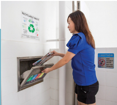
SEPARATE CHUTES FOR RECYCABLE WASTE
