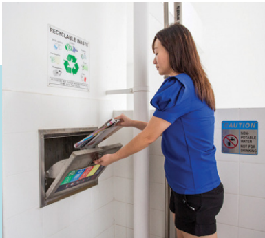
SEPARATE CHUTES FOR RECYCABLE WASTE
