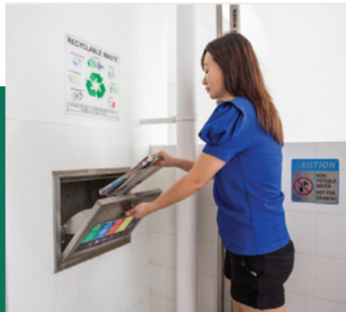
SEPARATE CHUTES FOR RECYCLABLE WASTE
